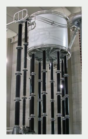
**SMOOTHING REACTOR** Smoothing reactor for HVDC application.
