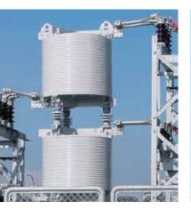
Filter reactors are used in conjunction with capacitor banks to form tuned harmonic filter circuits, or with capacitor banks and resistors to form broadband harmonic filter circuits.
