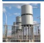
Reactors improve the overall efficiency of transmission and distribution systems through reduction of losses and fault current levels improving reliability and increasing transmission capacity.
