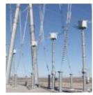
Line Traps form part of the Power Line Carrier communication scheme. It's function is to present a high impedance at the carrier frequency band while introducing negligible impedance at the power frequency.
